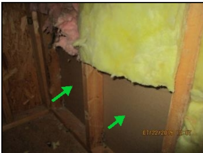
Wall insulation is missing.
