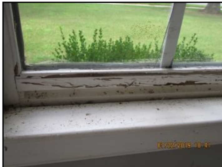
Garage window is broken and moisture damaged.
