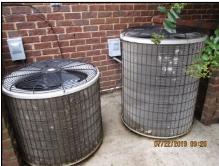
HVAC condensing units.
