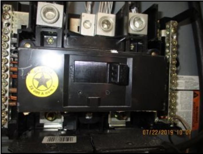
200 amp main electrical service disconnect.
