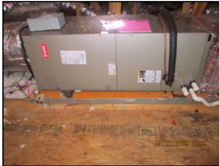
Air handler for second floor HVAC system.
