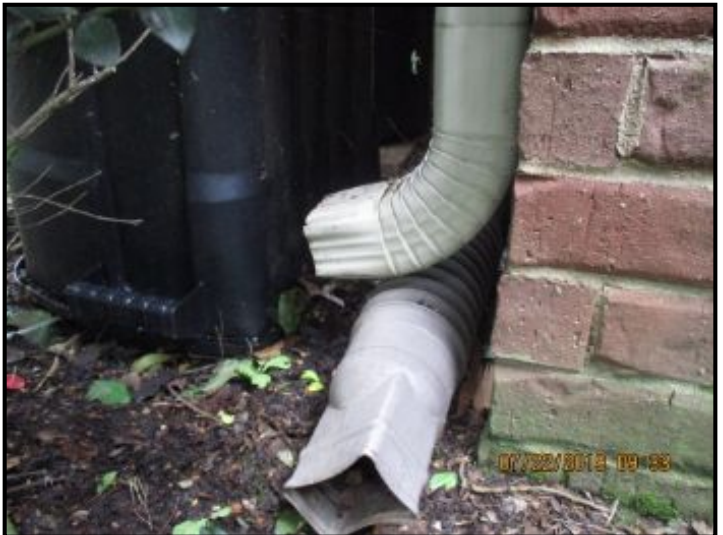
Down spouts need extensions to carry water away from the foundation.
