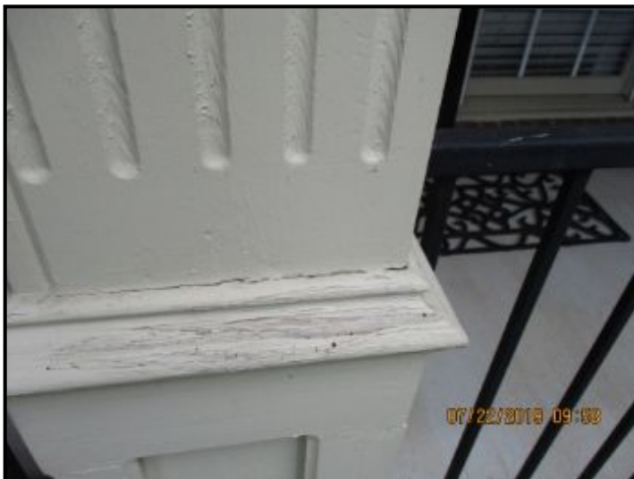
Cracking paint on columns.
