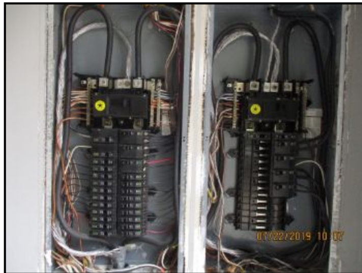
Main electrical service panels.
