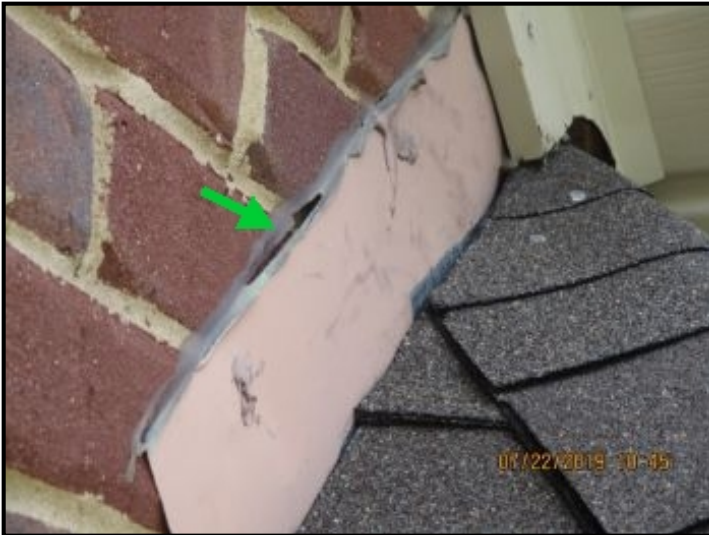
This flashing needs to be caulked.
