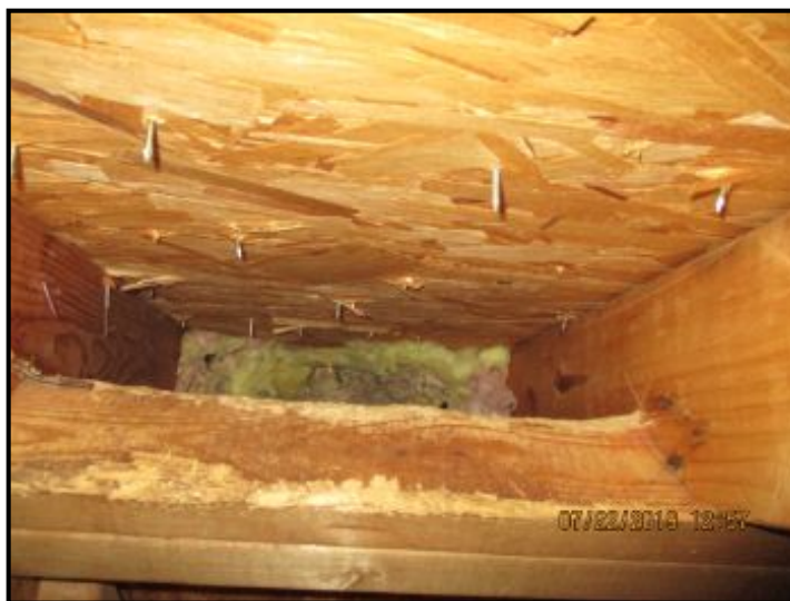
Rodent damage in bonus attic area.
