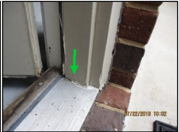
Patio door leaks at the threshold.
