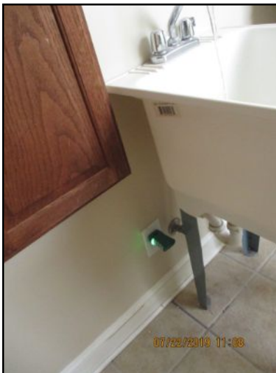
This receptacle need to be GFCI protected.
