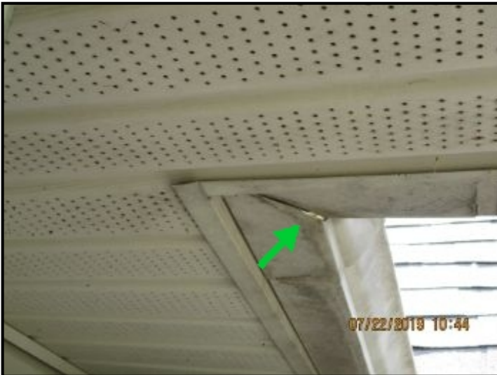
Leaking gutter seams and corners.
