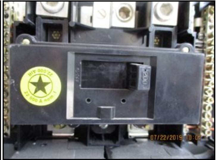
Main electrical service disconnect.
