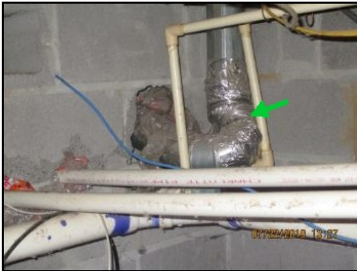
Flexible dryer vent pipe.
