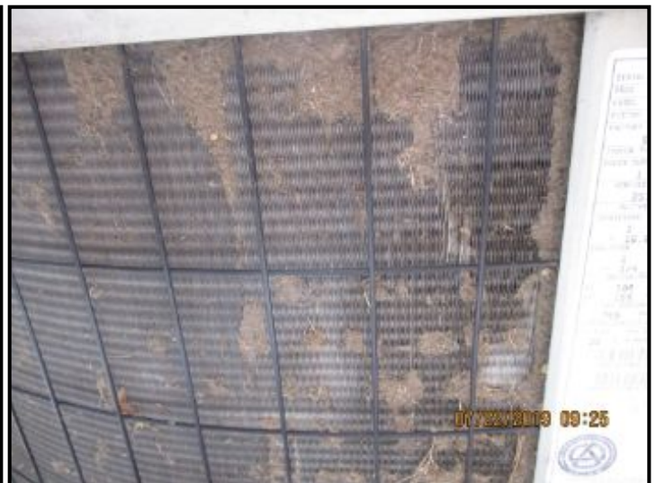
Condensing coils are dirty.
