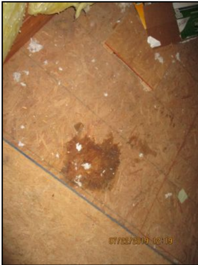
Condensate dripping on the structure.
