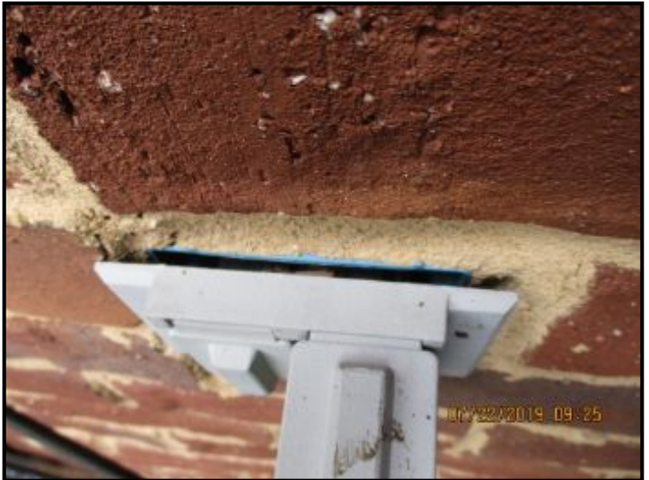
Loose exterior receptacle cover.
