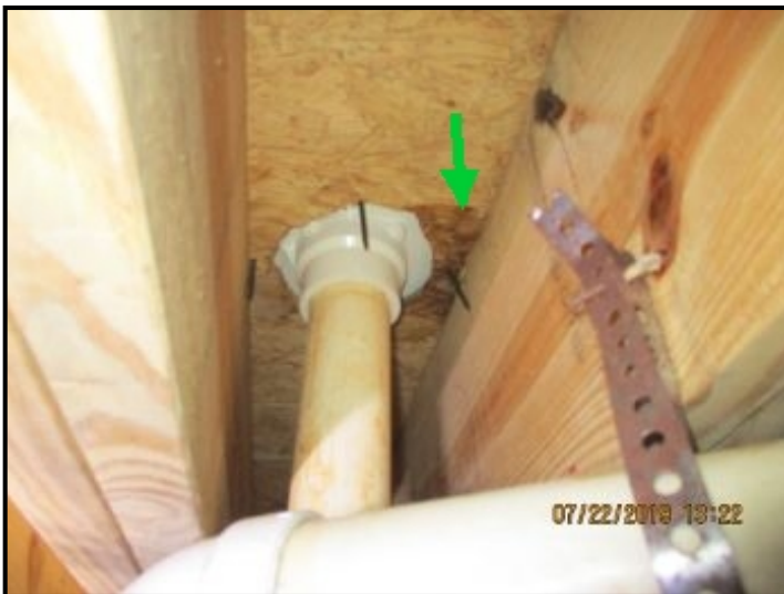
Master shower drain is leaking.
